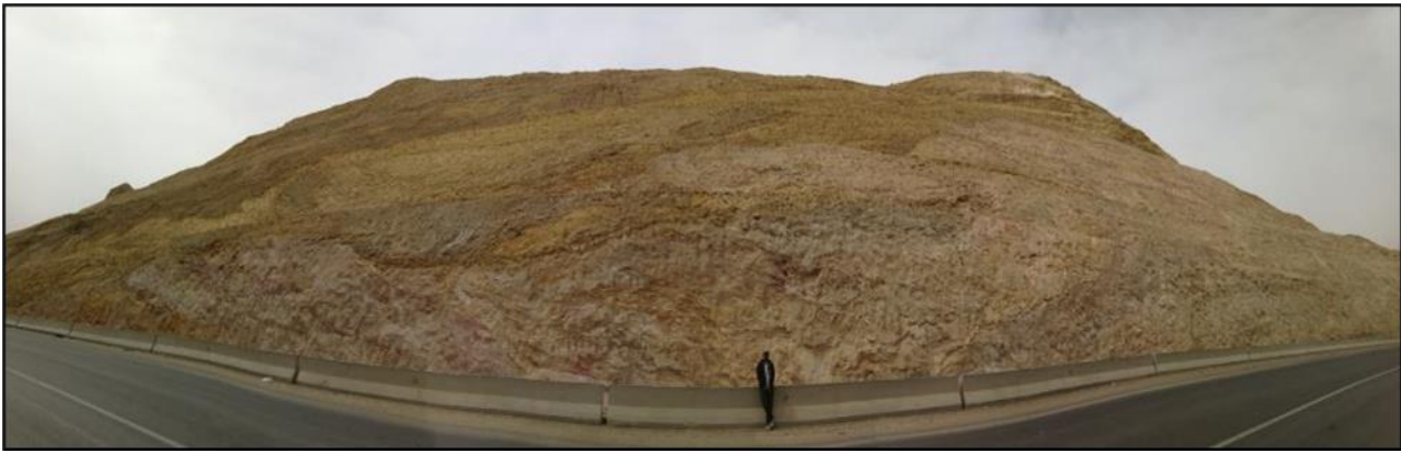
Fig. 5 Field panoramic view of the existing rock cut slope in different rock masses along station no. (4)
